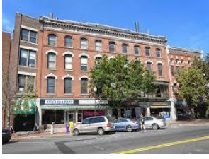
57school Street 413-772-0055 Greenfield, MA
